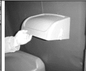
Note: When installing with Swish Tank, position paperguard bottom 2" above the top two dimples, mark and drill using holes in paperguard and rivet.
