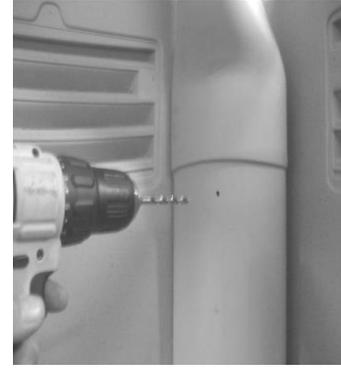
Using a silver colored expanding rivet PN 17436, attach the coat hook to the vent pipe.
